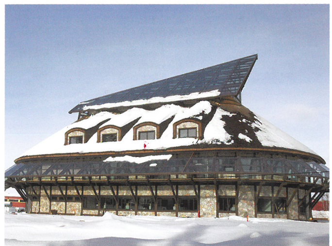
Biolan Oy, Eura, 2010. Triple-glazed insulating glass, 3 K A6(h)-15 Ar-K6(h)-15-(4(h)+JT22+4(h)), all tempered. Balcony ceilings: tempered laminated A6(h)+6(h)JT22. Railing glass: tempered laminated 6(h)+6(h) and 8(h)+8(h).
