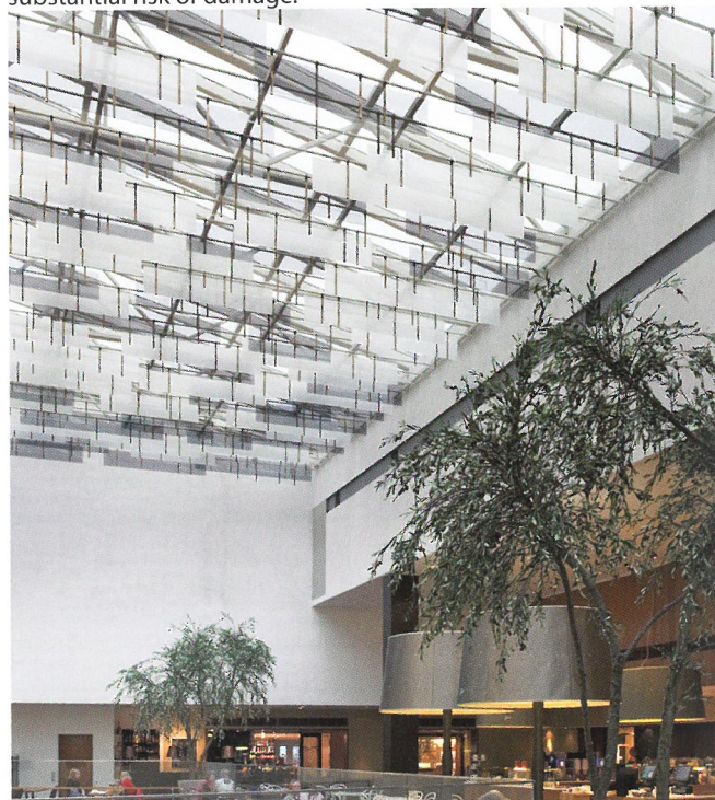
Stockmann Oy Helsinki, 2009. Artwork "Iiris" on restaurant's ceiling. Tempered and laminated, heat-soak tested glass 6+6 Optiwhite glass with various coloured interlayers, polished edges.
