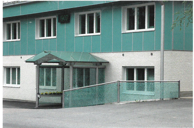
Offices of Jaakko-Tuote Oy. Upper section laminated spandrel glass 3+3, lower section tundra-patterned brick. JT Siruglass at entrance and railing.
