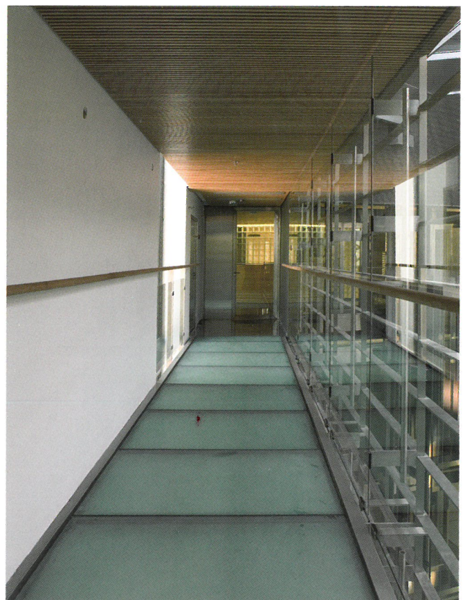
Parliament House extension, corridors' laminated floor glass 12+12+12, sandblasted.
